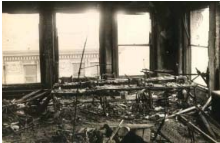
The ninth floor of the Asch Building after the fire. The building was fireproof and was subsequently renovated. The contents, however, were not fireproof. The remains of two of Triangle’s long work benches can be seen, revealing how closely the workers were packed together on the shop floor. The long drive shaft that simultaneously powered all the sewing machines on the bench can be seen under the closer bench.
